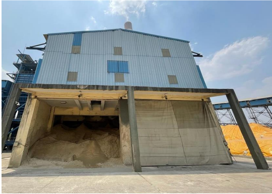
FIGURE 7: CURTAINS ON FGD STORAGE YARD
