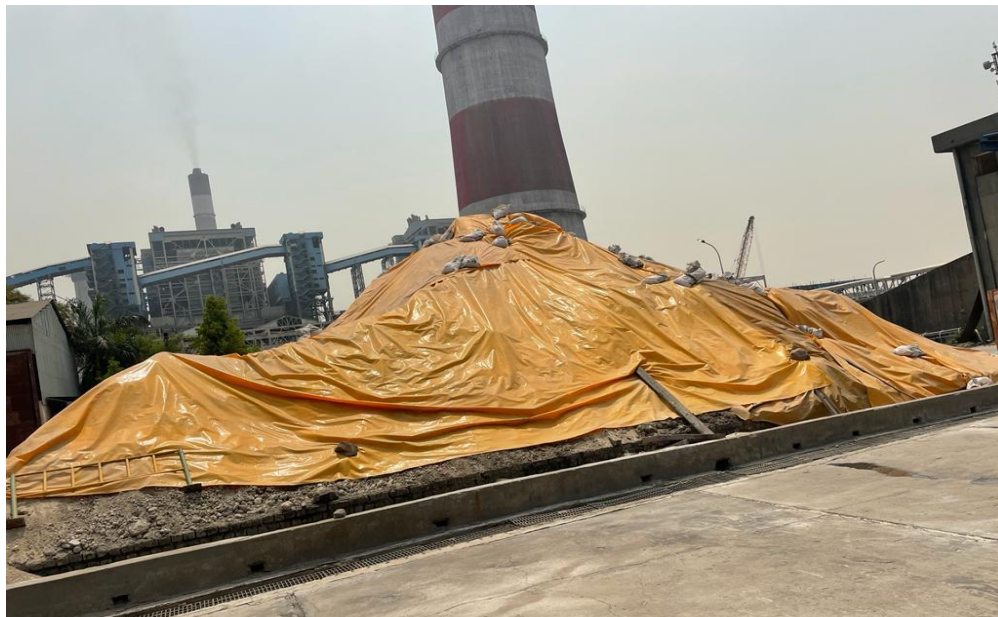
FIGURE 7: CURTAINS ON FGD STORAGE YARD
