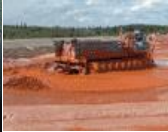
Figure 19: Dry Mud Stacking
