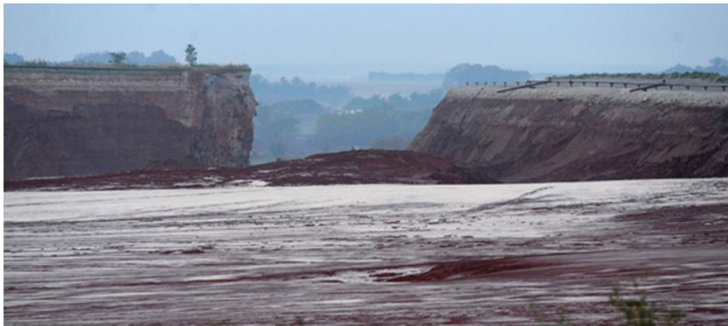
The West and the North Dam after the failure
