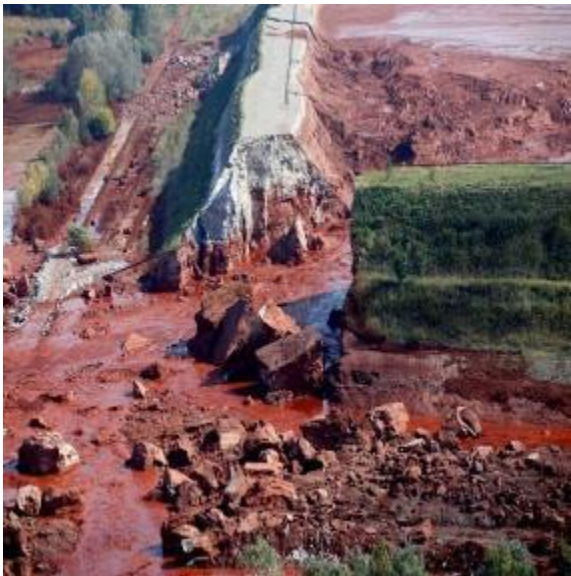
The West and the North Dam after the failure
