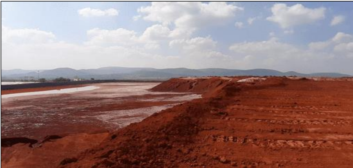
Red Mud Disposal Pond
