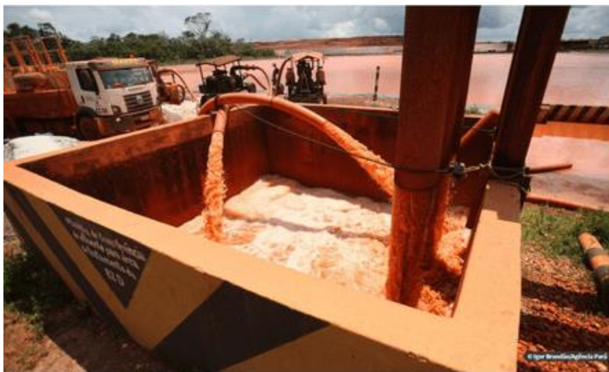
Figure 24: Image of the mixing box and area around during the flood situation
