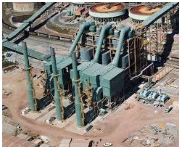
Gas Suspension (Fluid Bed) Calciners
